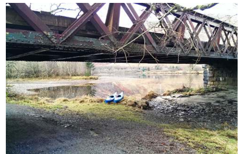
Railway bridge launch/landing point near Kilchurn Castle
